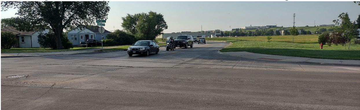
The intersection has north-south stop control and left turn lanes on north, east and west approaches, as well as a right turn lane on the east approach. The intersection experiences unacceptable delay and LOS under the existing 2023 PM peak conditions and is expected to continue to deteriorate through 2045 if no improvements are made.
