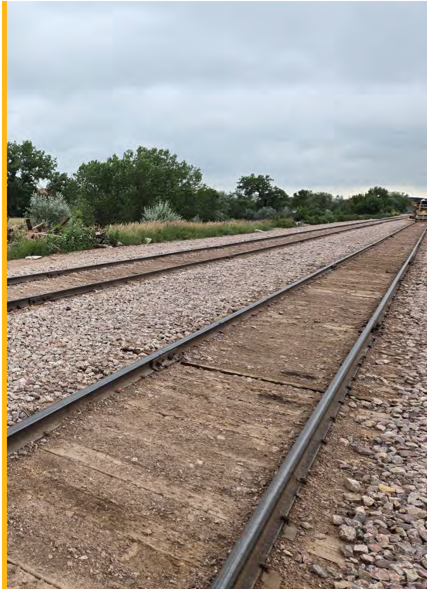
Figure 10: Railroad track at existing site
