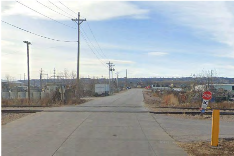
Figure 13: Culvert Street Private Crossing
