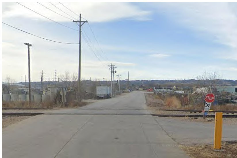
Figure 13: Culvert Street Private Crossing
