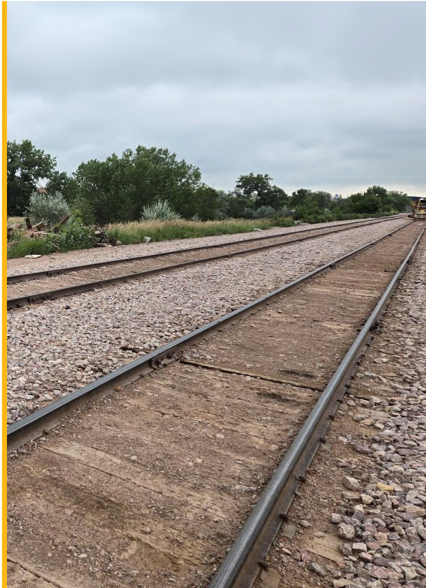
Figure 10: Railroad track at existing site
