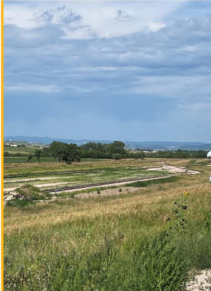
Figure 41: Existing track at Box Elder Candidate Site
